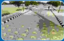
Interlocking Tiles Road
